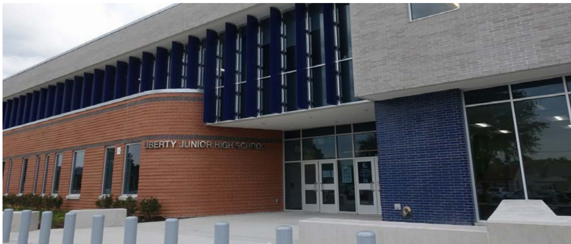
West entrance, used for student bus access and after-hours plays, sports and other events
