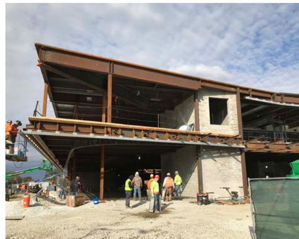
Structural steel at 18' cantilever at second level
