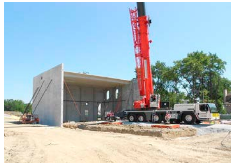
Erecting storm shelter envelope
