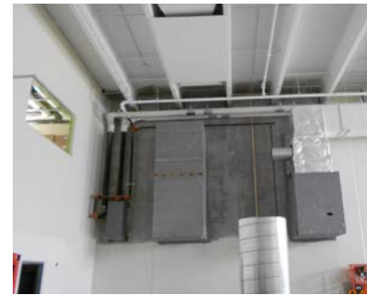
Steel shrouds at penetrations
