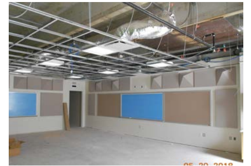
Music room with steel protection visible
