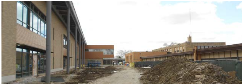
Construction photo showing new school with existing school beyond
